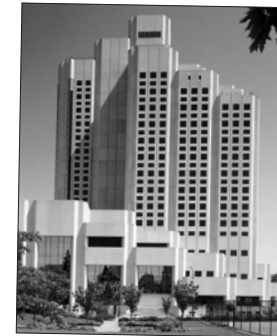
Laurel Pavilion, Vancouver General Hospital, 1982 Architect: David Rodgers (Thompson Berwick Pratt & Partners)
